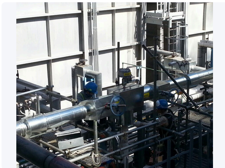
After: the Jetomat in its insulated housing, with its actuator, during installation.
